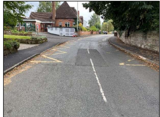
Figure 12: Bradford Road, Belbroughton
